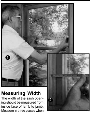
measuring the width. Top, bottom and middle. Report the smallest measurement taken.
